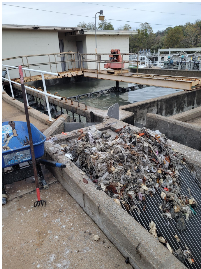
Non-organics captured at manual bar screen
